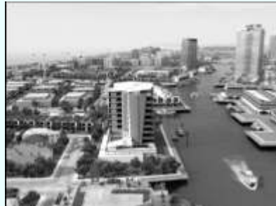
Fremantle island project.
